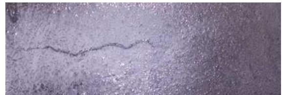
Fig. 3. Sample with crack
